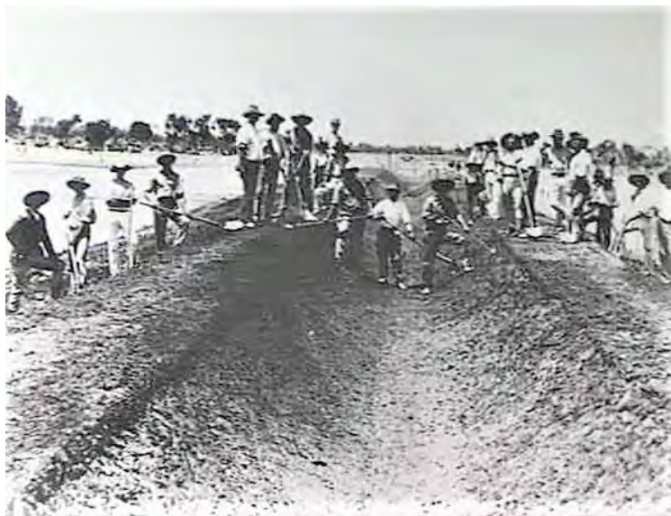
Building an irrigation channel at Renmark. Note that the heaviest earthmoving appliance in the image is a shovel. Image: State Library of South Australia, Catalogue number B53443.
