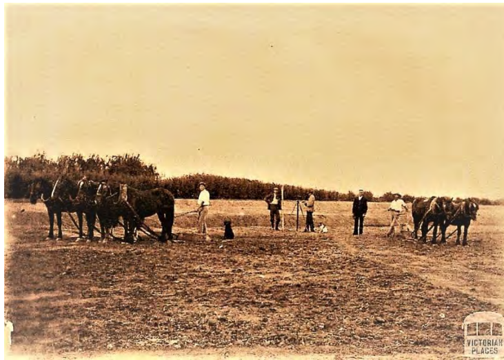
Taking levels for construction of irrigation channels at Mildura. Image: Victorian Places.
